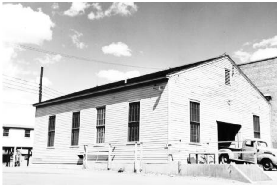
Technical Building Z. This shack was built for the Cockcroft-Walton accelerator in 1943.
