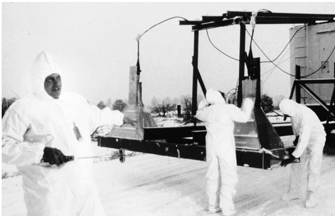
Ground-penetrating Radar Units. These units are effective at testing the integrity of shallowly buried fuel-storage tanks. Depth penetration is up to tens of meters in lossy soils and up to a kilometer under ice.
